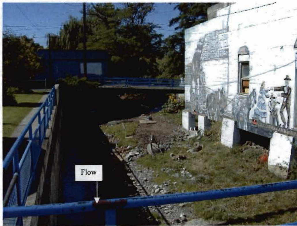
Photo No. 59 : View looks upstream (south) at the main stem of Birch Creek from Main St. bridge, showing building encroachment.
